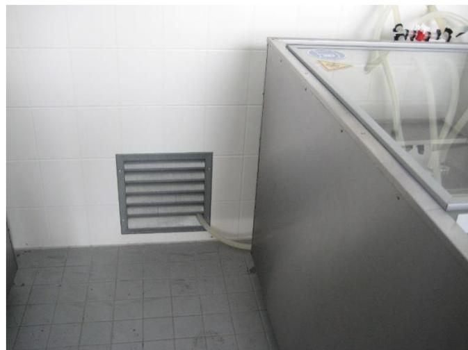
**Fig. 6: Room ventilation with a ventilation opening beside a freezer chest. As solvent vapours are heavier than air, it is advantageous to extract them close to ground level.**
