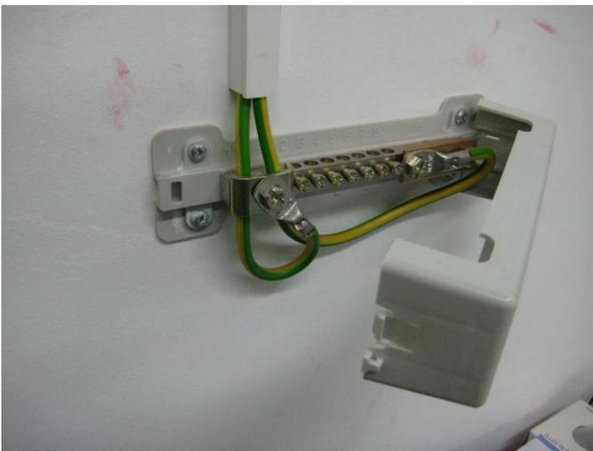
Fig. 8: Wall-mounted potential equalisation bar with several connection options.
