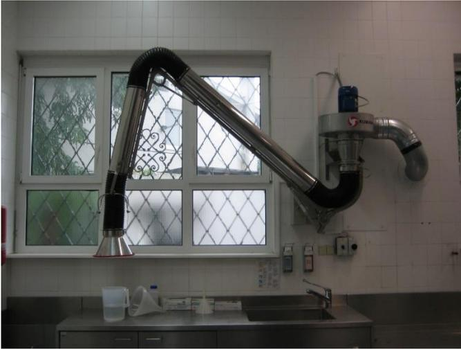
Fig. 7: Extraction arm with explosion-proof fan on top, offering workplace ventilation.
